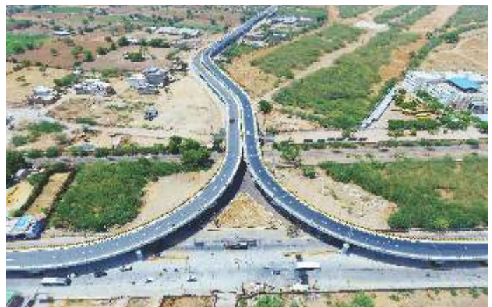
ROB at Jodhpur, Rajasthan
